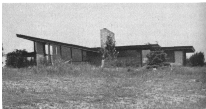
Fig. 7. Robert Levin house, Kalamazoo, Michigan, 1951. View from the south.
